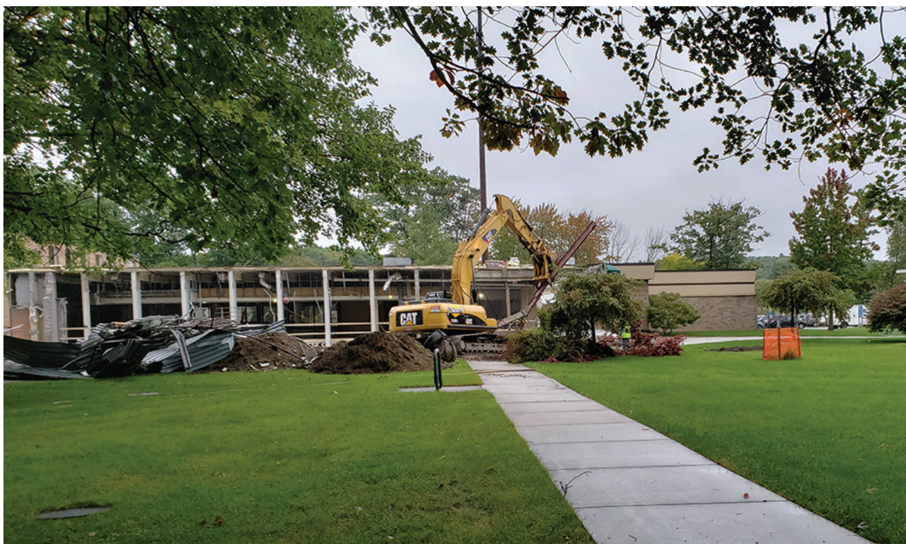
A bulldozer moves metal beams as a member of the crew hoses down the demolition site of West Hall on Oct. 3.
